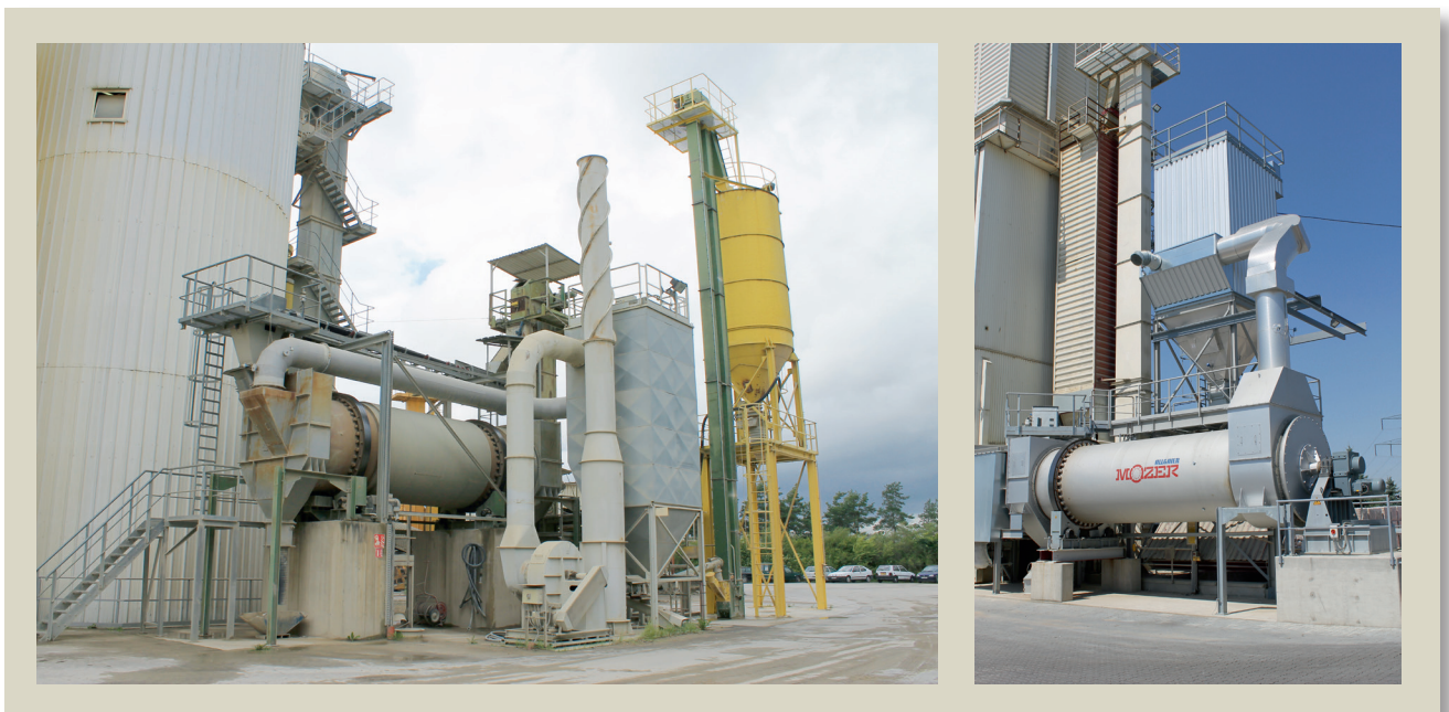
Figure 1: Dryer drum/cooler for sand
