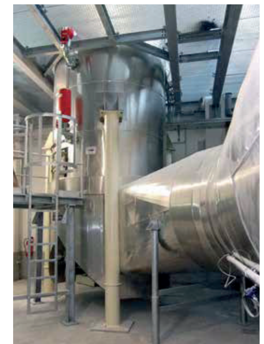
Dryer lower section with drying air inlet
